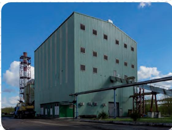
Since 2008, all bark and wood waste, together with sludge from treatment facilities, have been burned to obtain heat energy in a powerful boiler. The ash formed as a result of waste incineration is cooled and utilized without posing a threat of environmental pollution.
